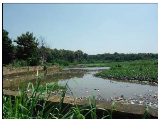
Plate 4.12: Solid Wastes and Siltation of Ogunpa Lake (Dandaru Reservoir)
