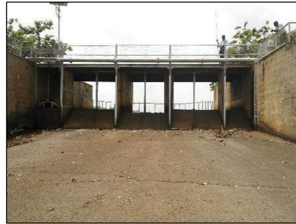
Plate 4.10: IITA Spillway and Downstream Channel
