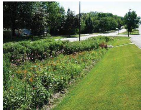
Plate 6.2: Swales Adjacent To Roads
