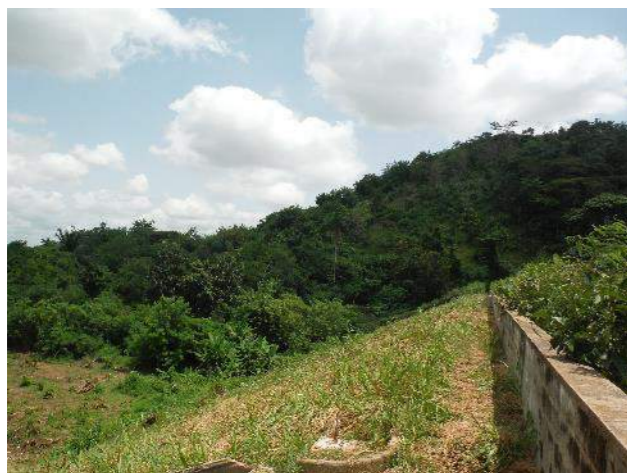
Plate 4.7: Parapet and Dam downstream embankment
