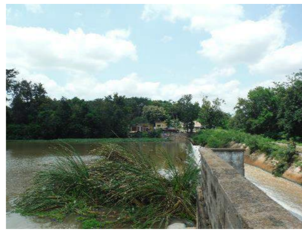
Plate 4.8: Dam's Parapet upstream and Spillway in the background
