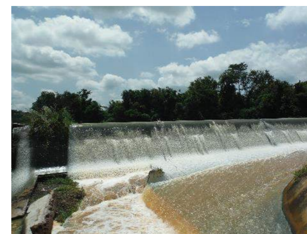
Plate 4.6: Spillway of Eleyele Dam
